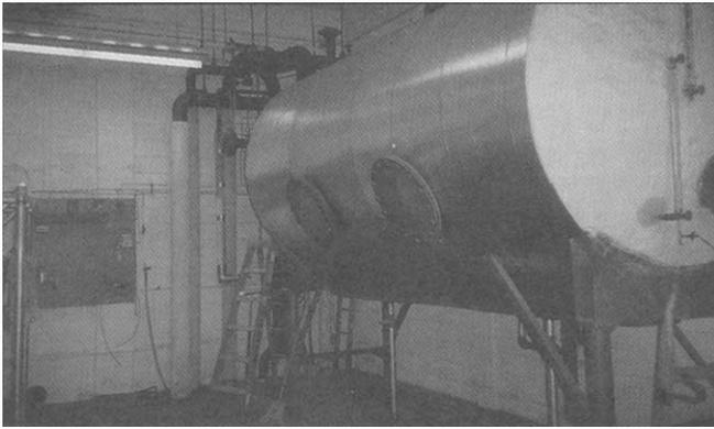
Figure 2. The 4000-gal (15-m<sup>3</sup>) settling tank located in the Heat Exchanger building.
