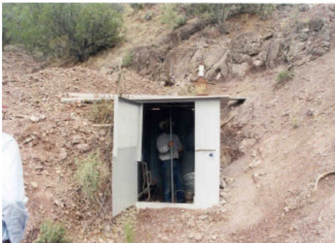
Photo 4. The Campbell 4 artesian geothermal well on the east bank of the Gila West Fork.
