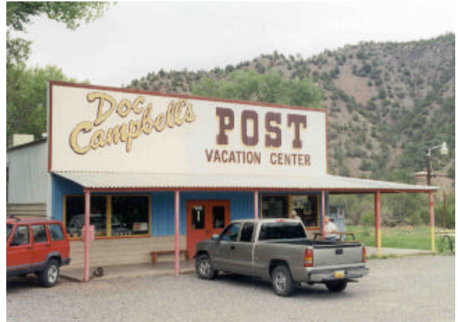
Photo 1. Doc Campbell's Store with geothermal floor heating.
