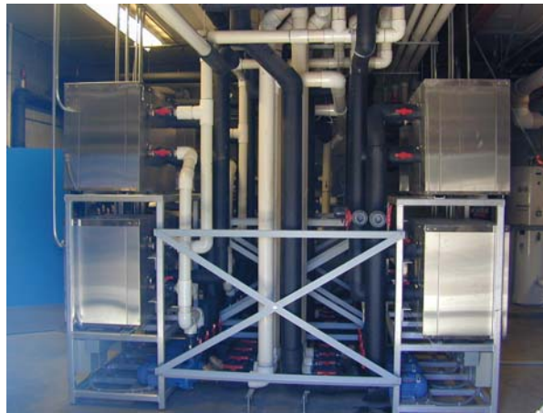
Figure 1. Eight low temperature water-to-water heat pumps provide approximately 84 tons of refrigeration at ice rink temperatures. The heat pumps reject heat either directly to a radiant floor heat system or to a horizontal earth loop.
