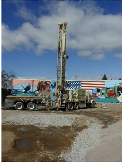
Figure 2. Photograph of drilling activities
